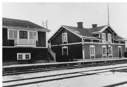
Jakobsbergs station. Foto: Joel Cardell.
